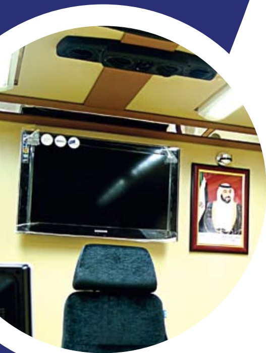
▲ 2 Aircondition Units and LCD Television for Office
