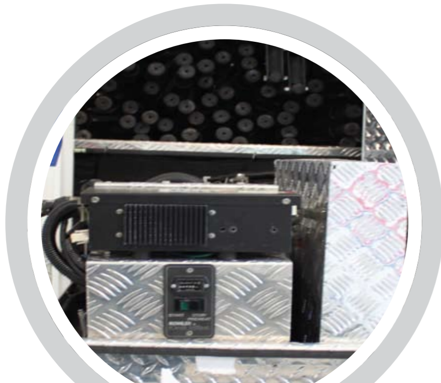
◀ Generator and Safety Equipments
